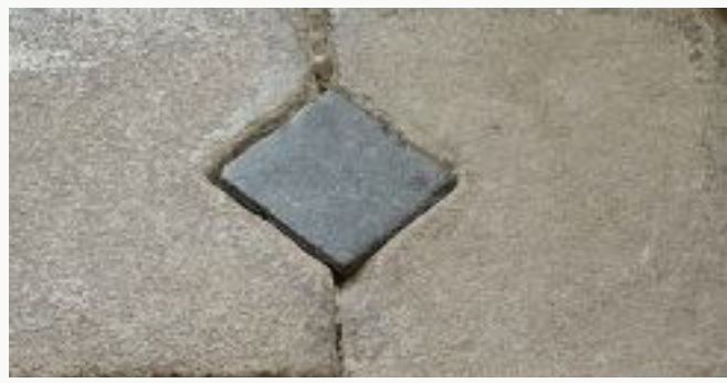
Door Jamb Threshold Piece with Beige Threshold and Grey Center 2"x2" Diamond
